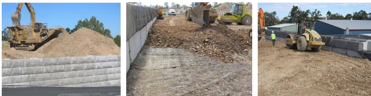
Figure 8: Construction processes of adopting in-situ materials
